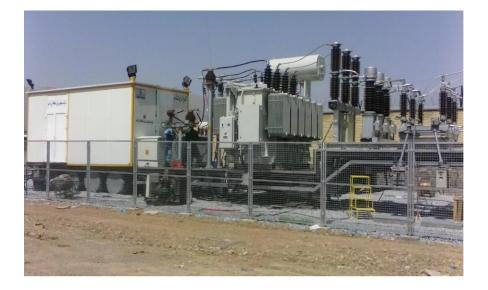
Mounted on skids, semi-trailers, trailers or in a container for rail and road transportation, the substations come as complete assemblies that are ready to connect. LTC ensures that the solution complies with the local grid code as well as the requirements posed by existing transformers that are running in parallel. Careful clarification of local transportation needs and choice of the truck ensures a smooth onsite delivery as well as easy mobility.
